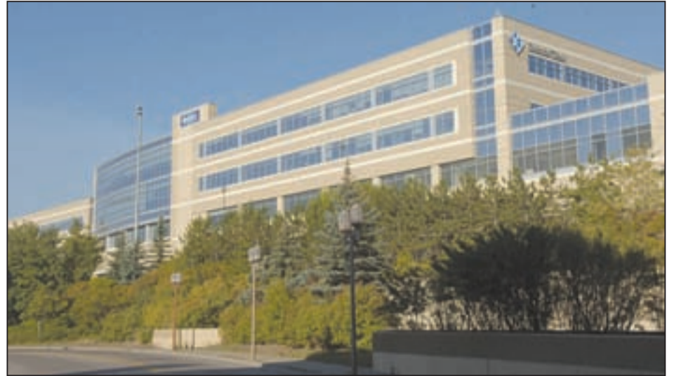
SMDC Health System's Duluth Clinic First Street Building is the largest health care facility in the country to receive a LEED-gold certification. The care center opened in April 2006, and received its gold rating in January from the U.S. Green Building Council. (Photo courtesy of Kim Kaiser at SMDC Health System)
